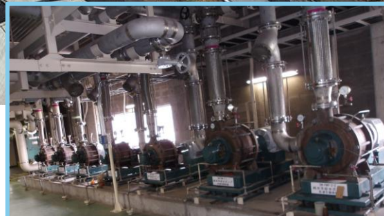
Various cooling pumps (primary and backup) and heat exchangers
