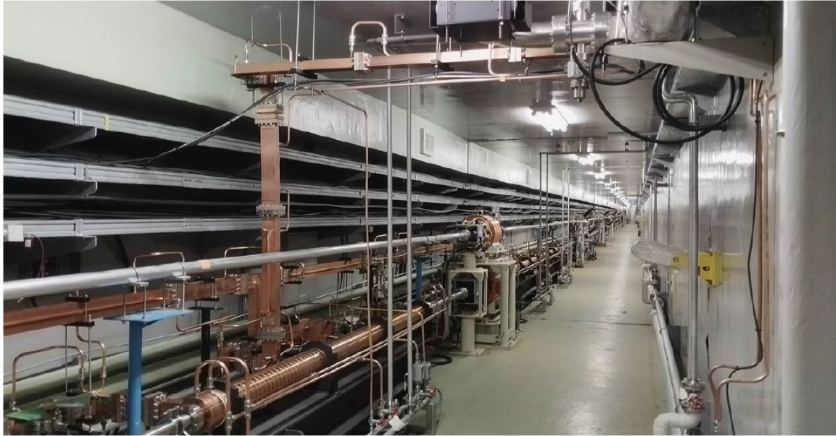
Four 3-m S-band accelerating structure
