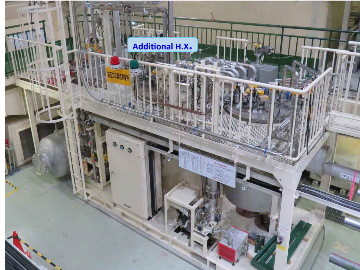
QCS-R Helium refrigerator and sub-cooler
