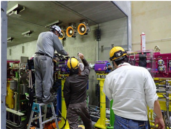
Alignment of magnets
