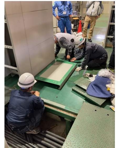
Reinforcement with steel to install the racks over the cable pits.
