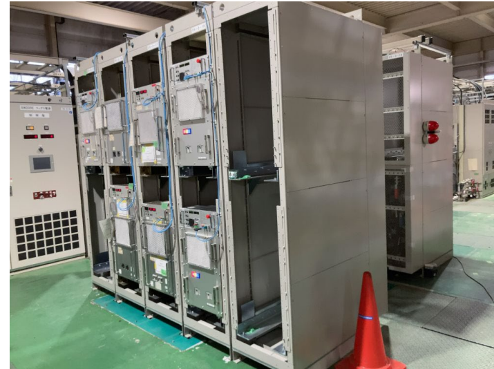
Additional breakers were added to the distribution board.
