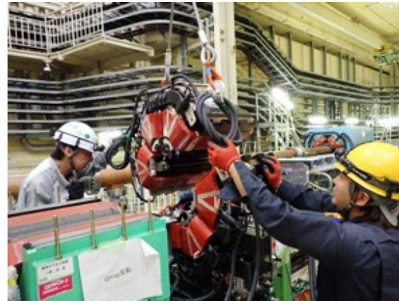
Installation of SNAP
