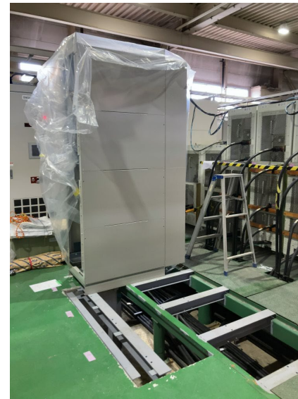
Reinforcement with steel to install the racks over the cable pits.
