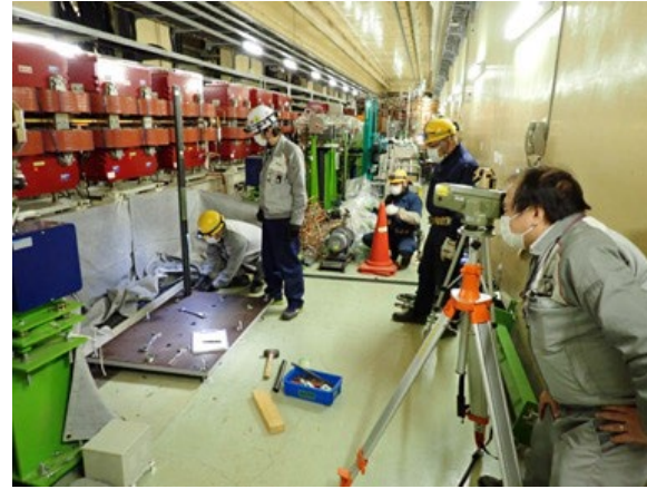
Production and alignment new baseplate
