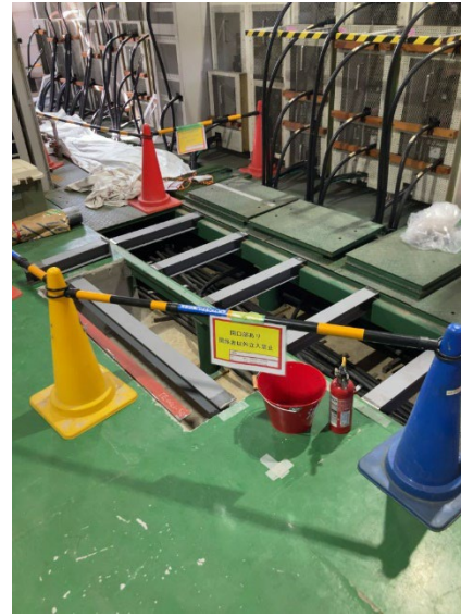
Reinforcement with steel to install the racks over the cable pits.
