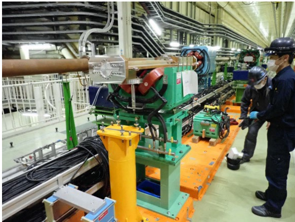
Installation beam chamber
